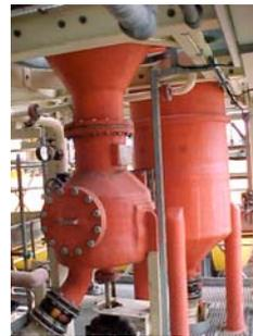
**Begg Cousland Venturi + Cyclone system in U.K. removing HCl mist and TiO<sub>2</sub> particulate.**
