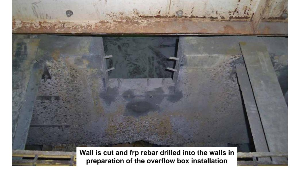
Prepping the overflow box exterior mold
